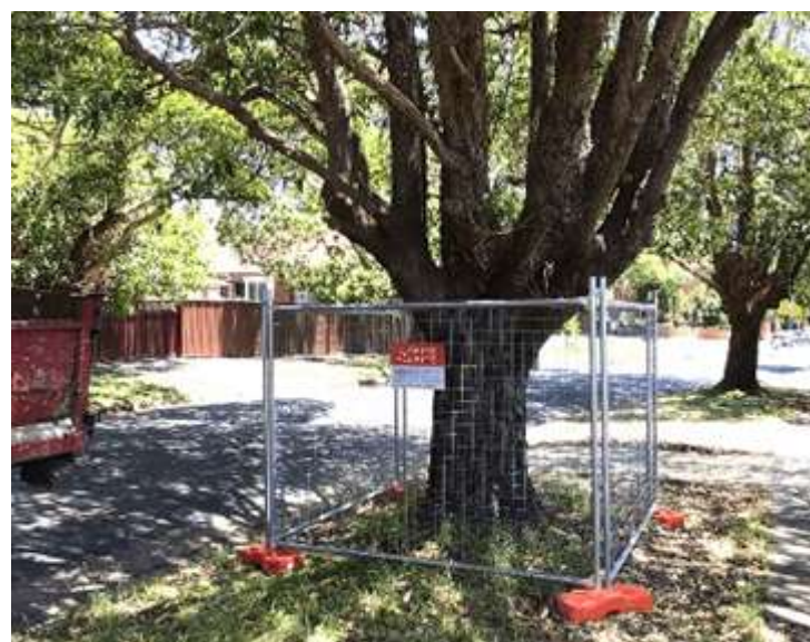
Figure 13– Examples of tree protection fencing.
