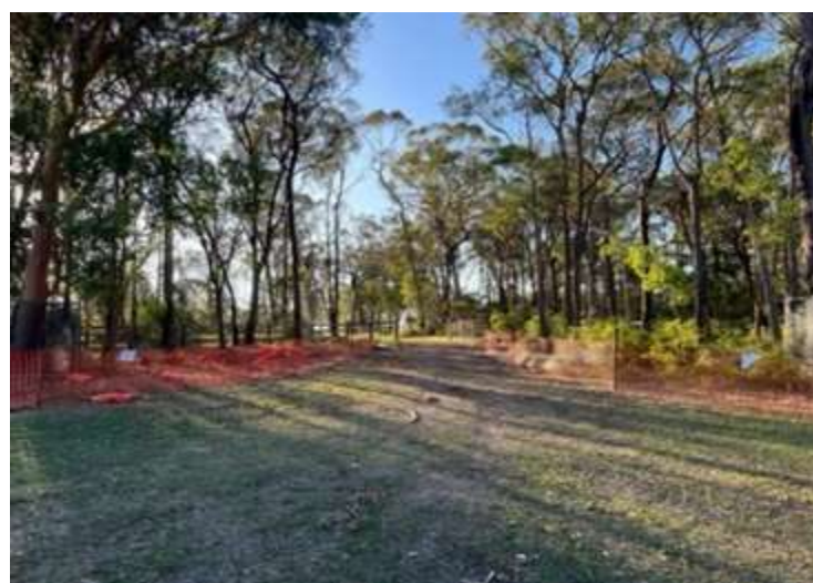
Figure 14-Webbing tree protection fencing.
