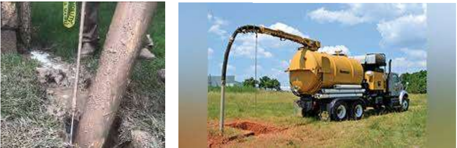
Figure 8 - Vacuuming. Figure 9 - Examples of Vacuum truck required. Source photos 4,5,6 and 7 TREX service excavations. Website
