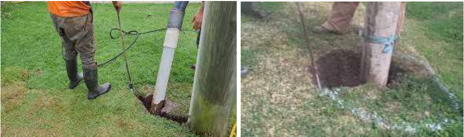
Figure 6 - Examples of Hydro-vacuum excava Figure 7- Hydro-vacuum excavation.
